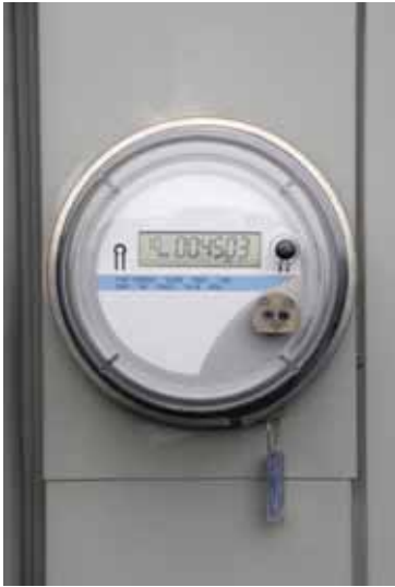
Smart meters, which enable two-way communications between power companies and consumers, are an essential component of the smart grid.
